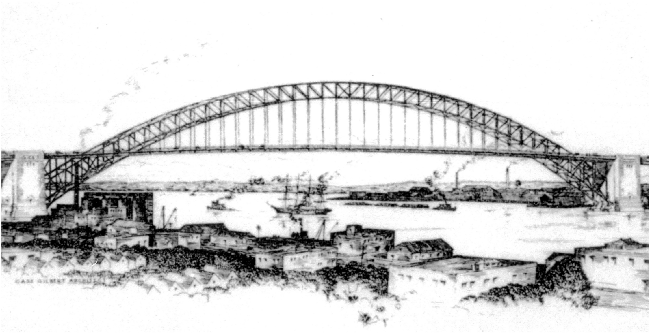
Cass Gilbert, Othmar Ammann: Bayonne Bridge, New York/New Jersey, 1931
