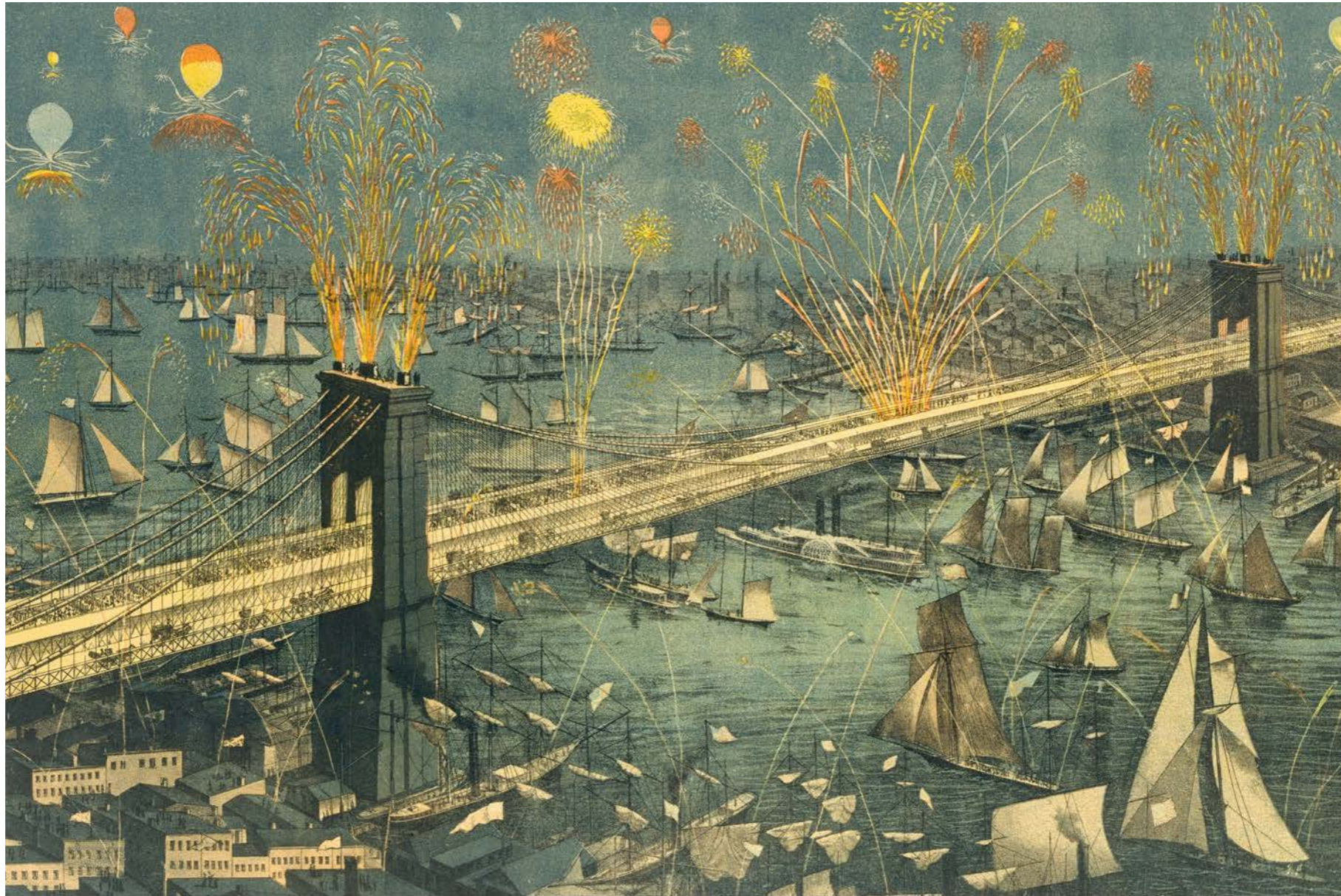
John August Roebling: Brooklyn Bridge, New York, 1883
