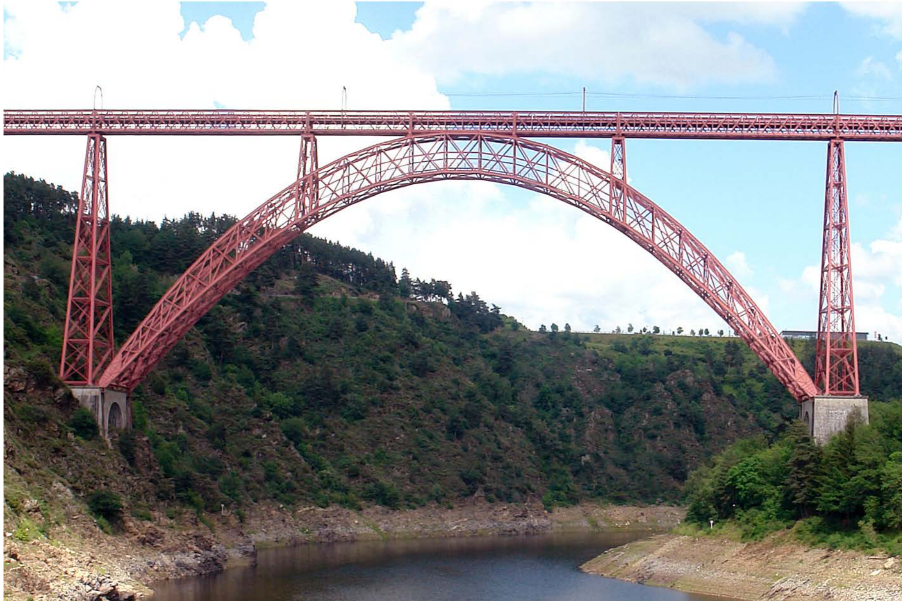
Gustave Eiffel, Maurice Koechlin, Léon Boyer: Garabit Viadukt, Ruynes, 1884
