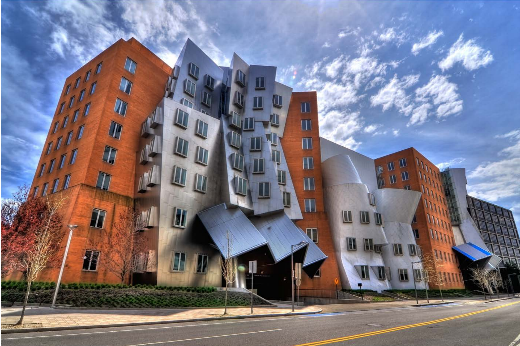
Frank Gehry, John A. Martin: Ray and Maria Stata Center, MIT, Cambridge, Massachusetts, 2004
