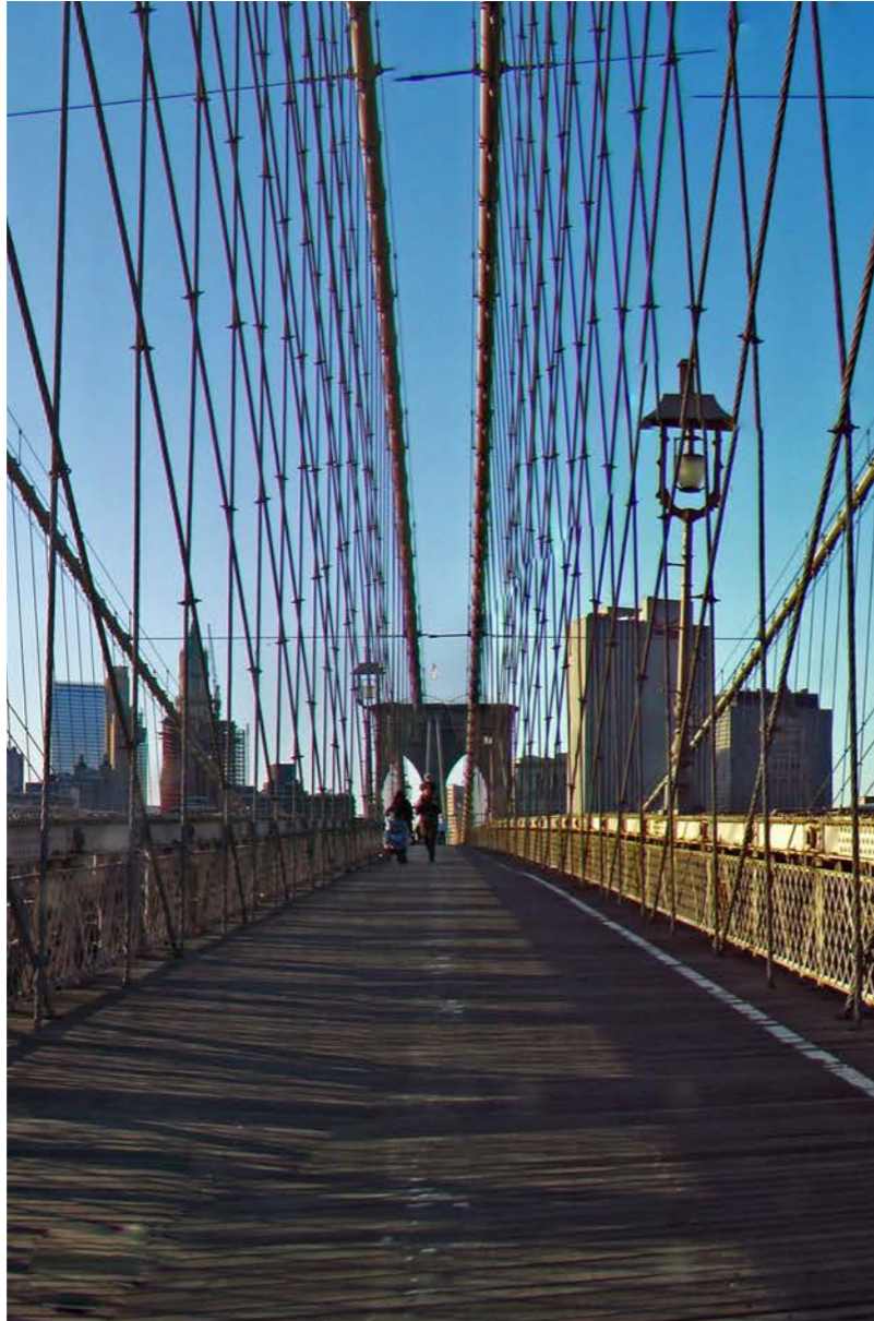
John August Roebling: Brooklyn Bridge, New York, 1883
