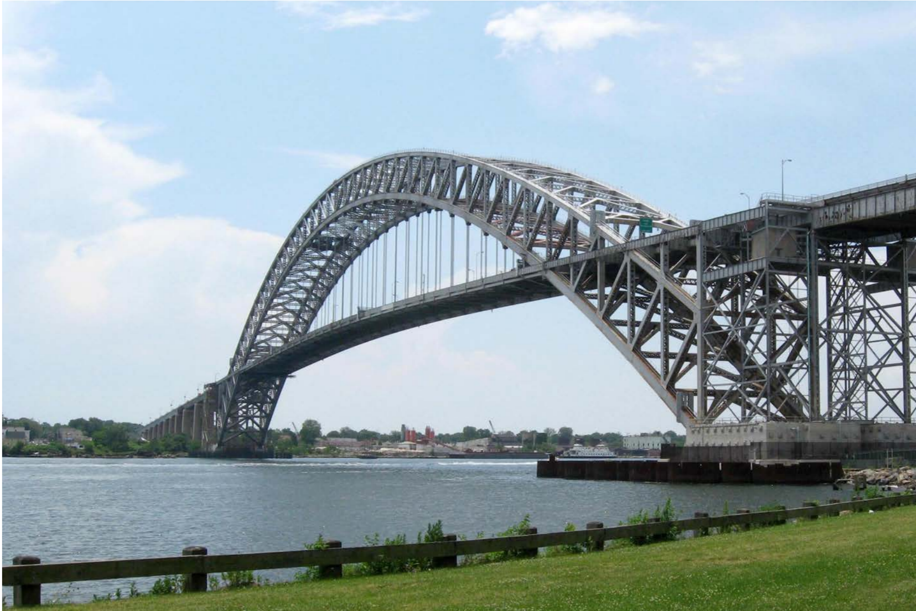
Cass Gilbert, Othmar Ammann: Bayonne Bridge, New York/New Jersey, 1931
