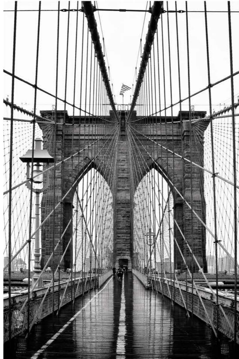
John August Roebling: Brooklyn Bridge, New York, 1883
